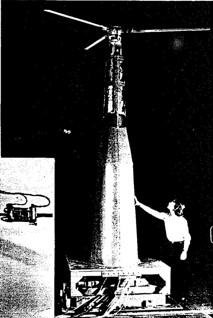
Fig.2 Upper rotor shaft assembly
