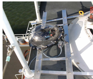
Figure 28. External installation of the video camera
