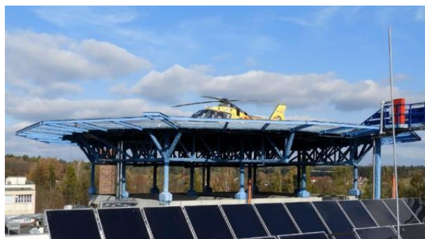
Fig. 1. Elevated helipad in hospital in Olsztyn, Poland
