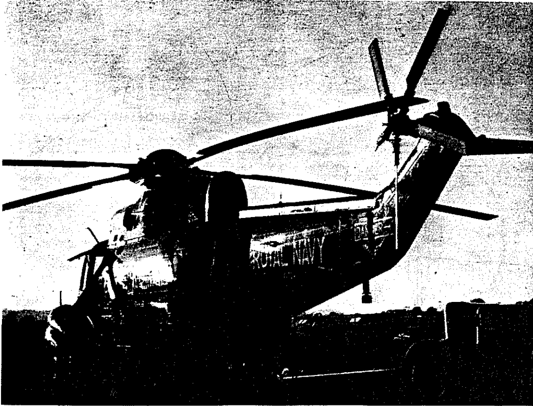
FIG. 5. SEA KING WITH CAMBERED TAIL ROTOR
