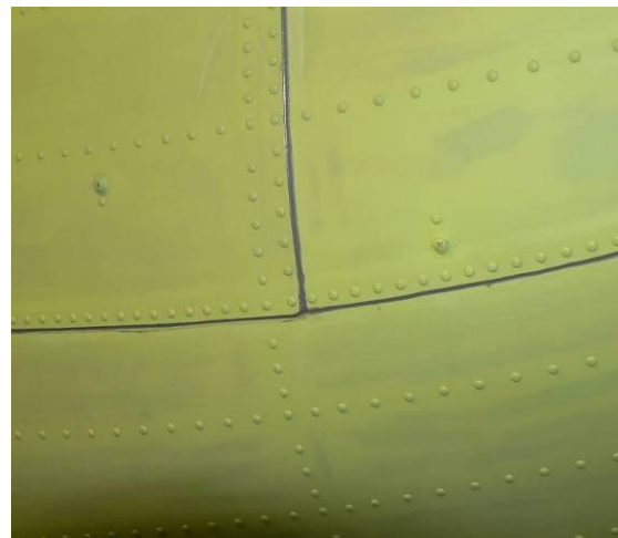
Figure 9, Shell, typical riveted technology
