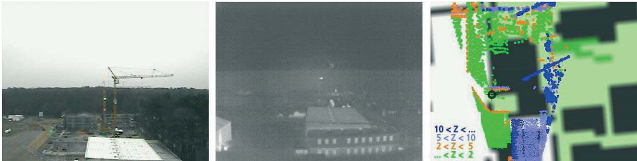
Fig. 7. View from a telemetry tower at Braunschweig airport onto a construction site of a new hangar. Left: color camera, center: IR camera, right: Lidar data (HELLAS). The Lidar data are overlaid onto a map display of the site's location. Certain height differences between Lidar measurements and terrain altitude are coded with different colors.
