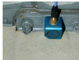
Figure 7. Detail view of the error sensor located inside the cabin just under the rear strut attachment point.
