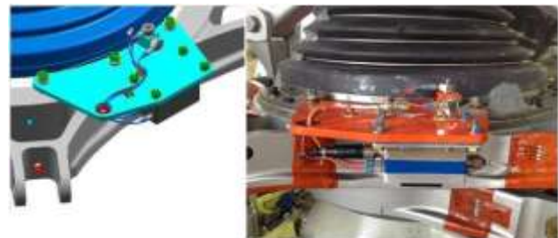
Figure 8: WSN Installation on AW139 Rotating Swashplate
