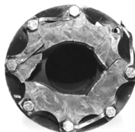
Figure 3: Plan view showing the fractured flange still attached to Shaft Section
