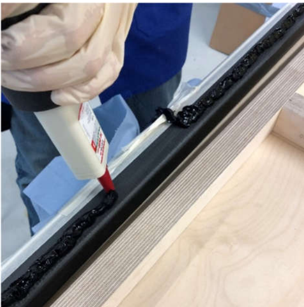
Figure 5 Application of paste adhesive on the CFRP frame of the canopy demonstrator [16]
