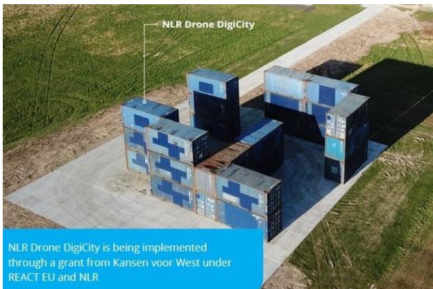
Figure 1: Picture of NLR Drone DigiCity
